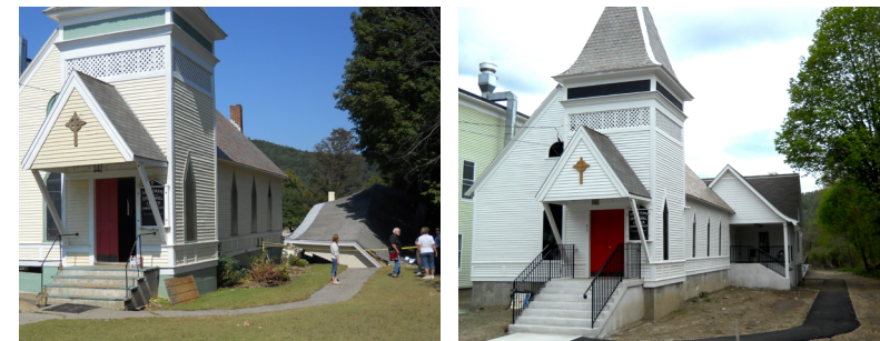
Left: Collapsed hall after Hurricane Irene Right: Hall rebuilt after hurricane damage
